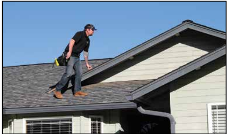
Matt Worthy performs a roof inspection.
