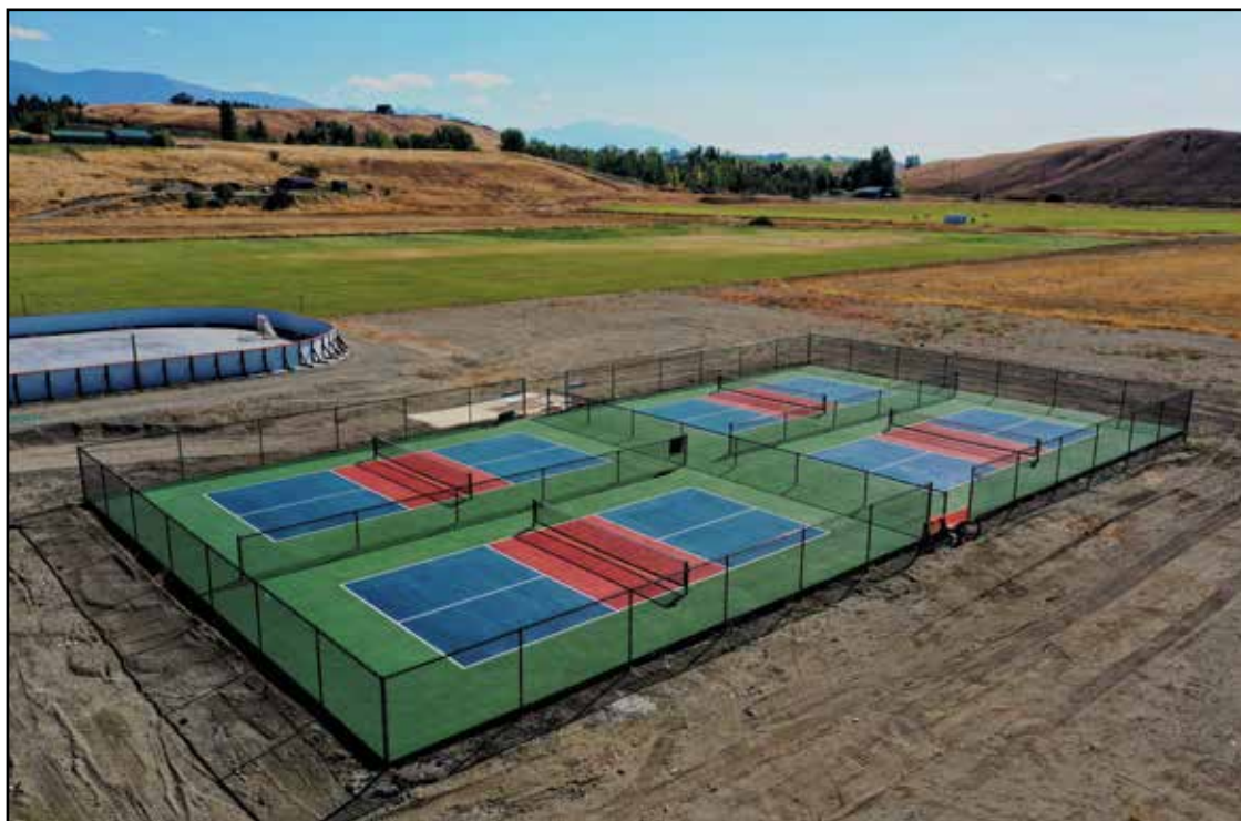
New pickleball courts.
